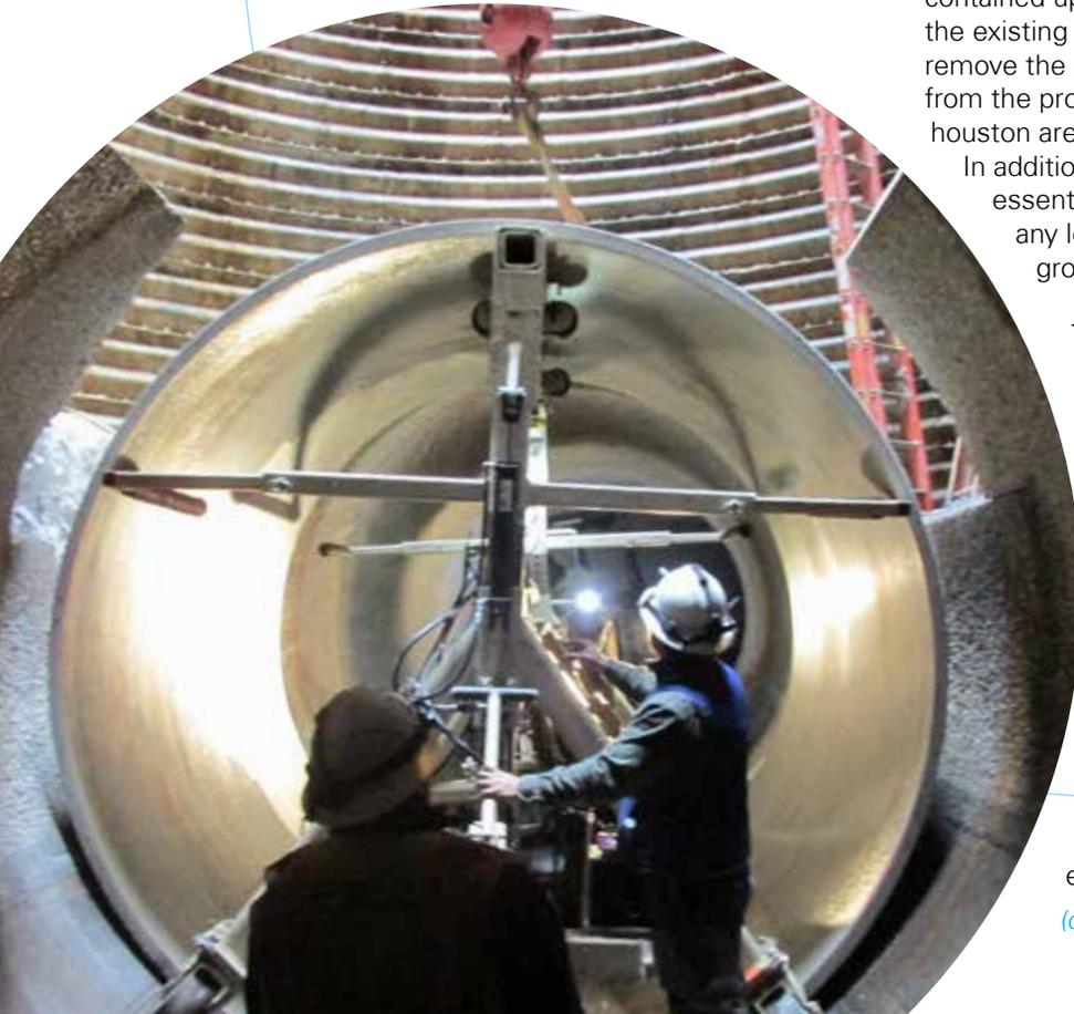
Short segments of CCFRPM pipe were manufactured by HOBAS Pipe USA to facilitate assembly into the existing curved host.
